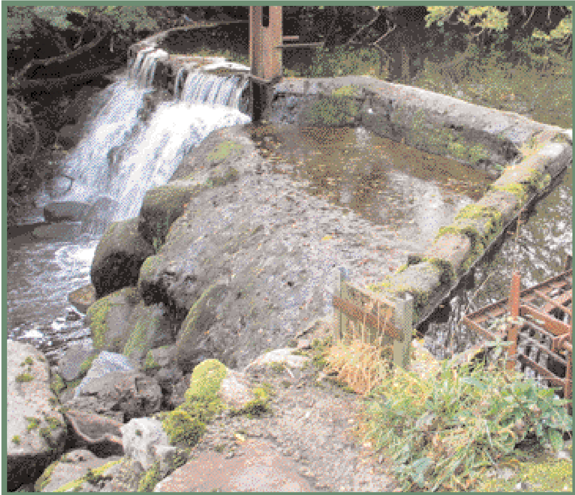
Impoundments created to divert water can block the upstream migration of salmon
